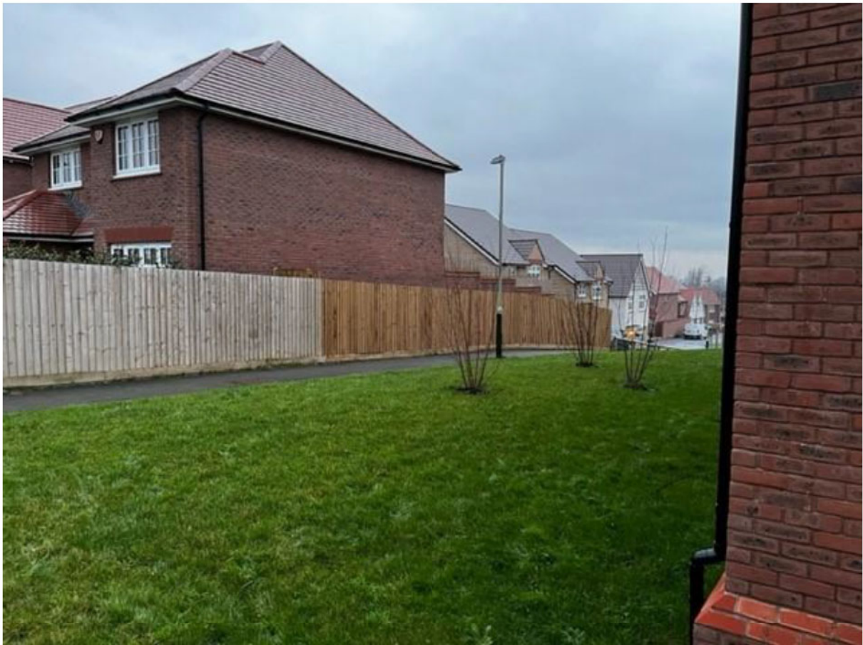
Photograph 3 The new fence next to the old fence installed by the contractors
