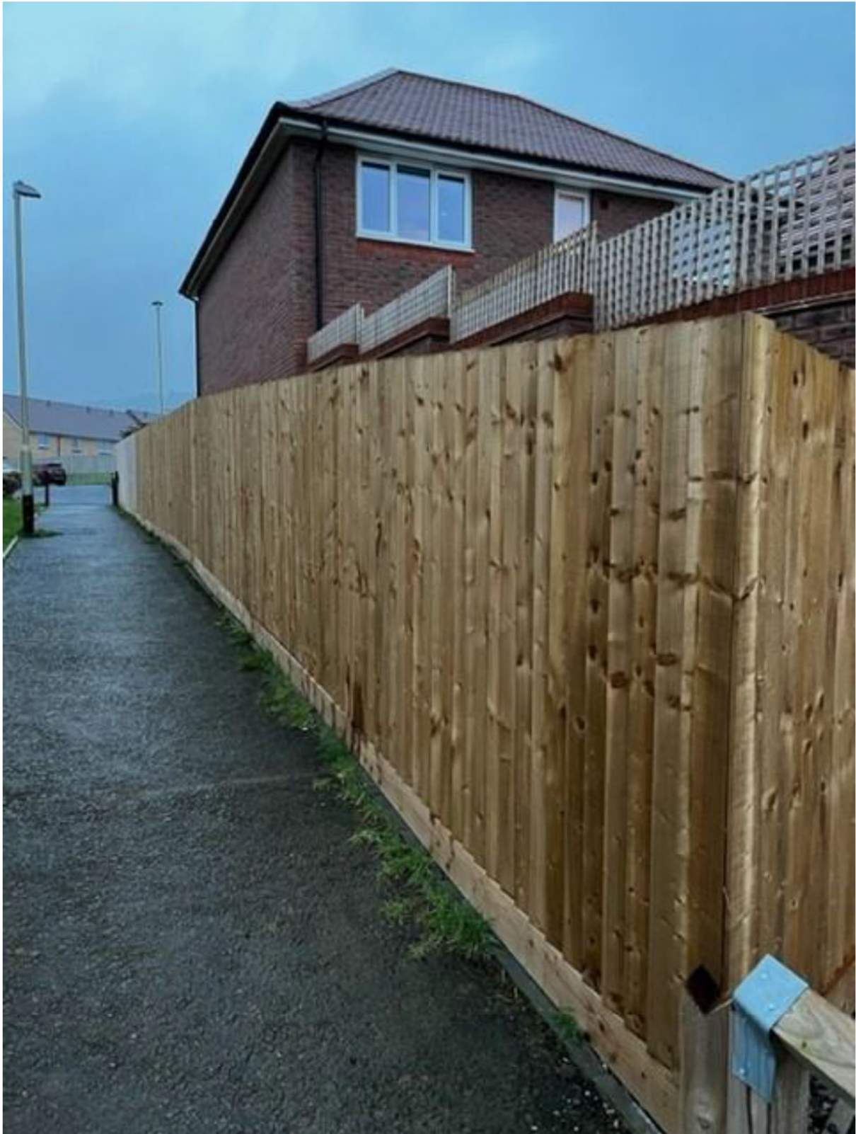
Photograph 2: The 1.8m high fence adjacent to the public footpath
